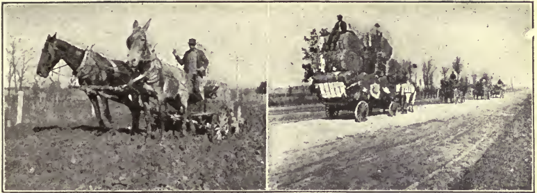
LIMIT OF TWO-HORSE TEAM OVER TWELVE BALES OF COTTON ON A BAD ROAD—TWO BALES OF COTTON MACADAM ROAD
